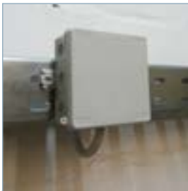
The EDV are suitable for installations at the long holes of the cable track. See page 22.
