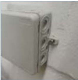
Classic fixture by screws and dowels.
